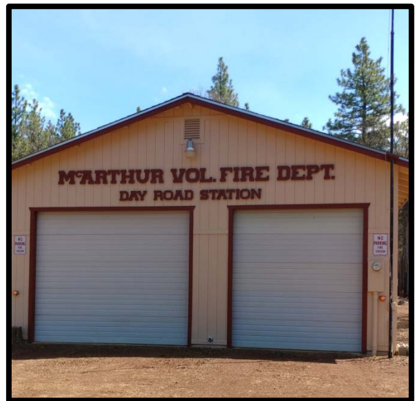
FIGURE 4– McArthur Fire Substation in Day
