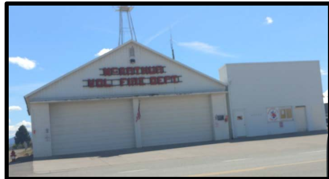
FIGURE 3– McArthur Volunteer Fire Department Main Station
